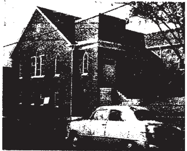
JUST FINISHED —The congregation of North Knoxville Baptist Church will hold its first worship service in its new $100,000 plant at 217 West Oldham Avenue tomorrow and have open house Nov. 28. The church was organized in 1930. The Rev. Kerr Wolfenbarger has been pastor 10 years.
